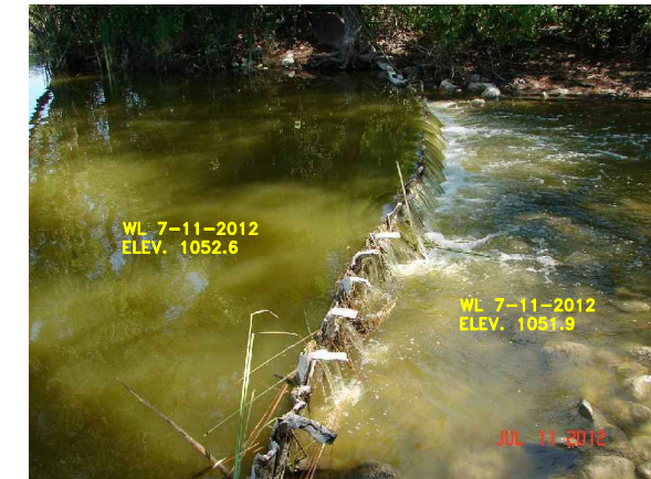
LOOKING EAST EXISTING SHEET PILE STR.
