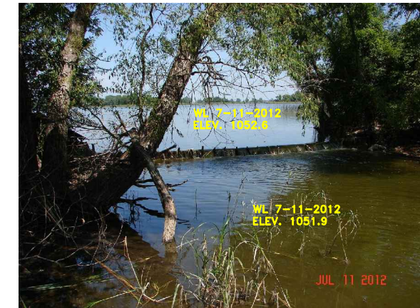
LOOKING NORTH EXISTING SHEET PILE STR.
