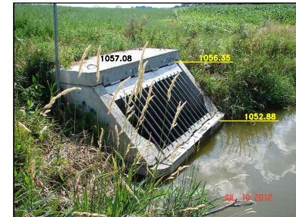
LOOKING SW CTY HWY STR.
